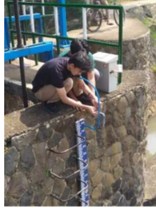
Fig. 13. Process installation sensor JSN-SR04.
