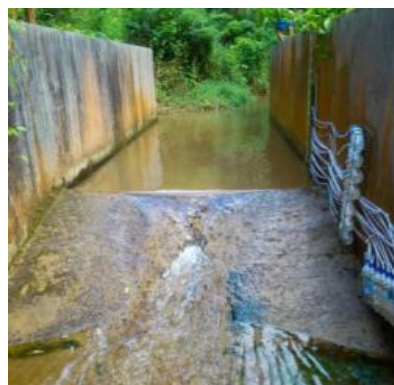
Gambar 2. SPAS Tipe Triangular Flat V-Weir di Sub-DAS Gajah Mungkur
